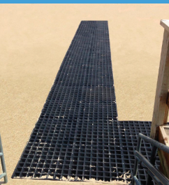
install access-a-mat tiles
